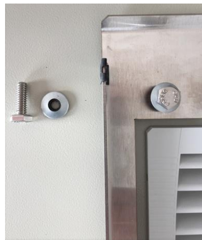
Figure 10: fasten 4x bolts for main frame
