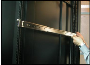
9. Secure the front end of the rail with two rack screws.
