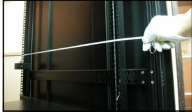
5. Take two pieces of rack rail, consisting of the middle piece with the pre-installed rear end, and one front end (left or right).
